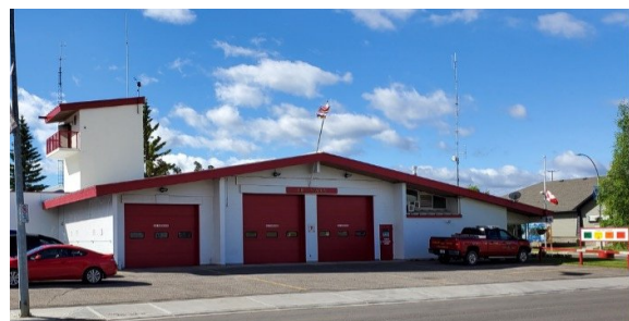
Figure 33: Tumbler Ridge fire Station
