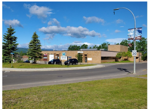
Figure 16: TR health care centre in the downtown core
