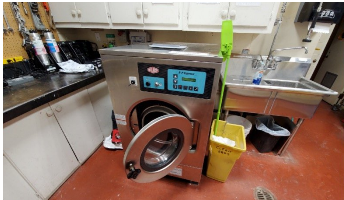
Figure 32: Tumbler Ridge FD extractor installed in work/service area.
