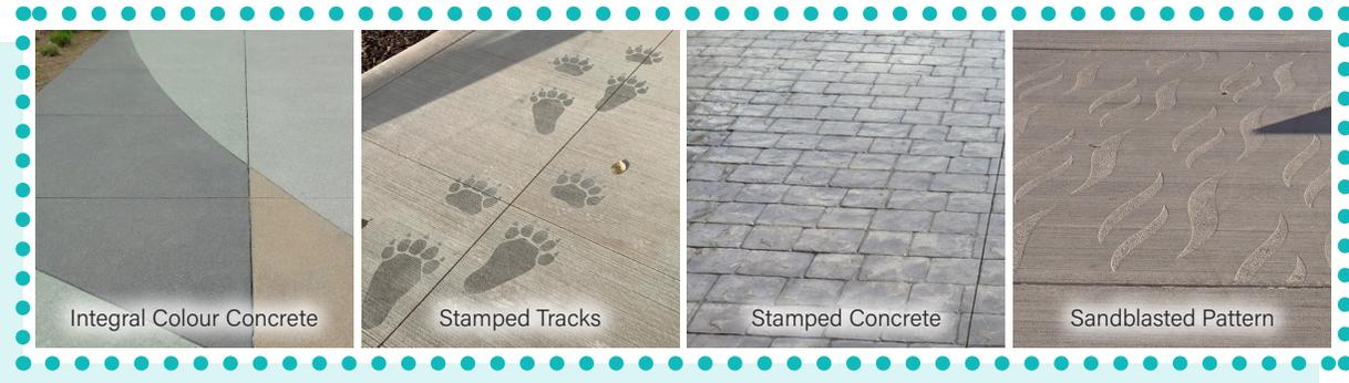
**Figure 15: Examples of different concrete surface treatments**
